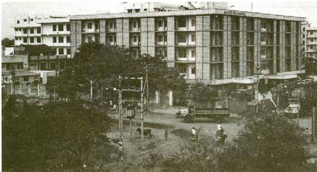
The new out-patient wing seen behind the main paying hospital
